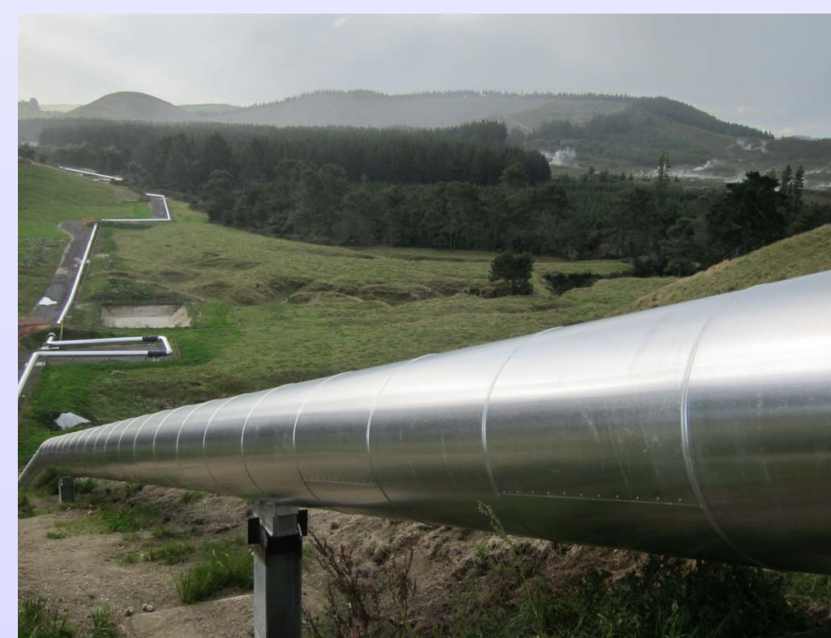
Figure 3. Brine transport pipe system.
